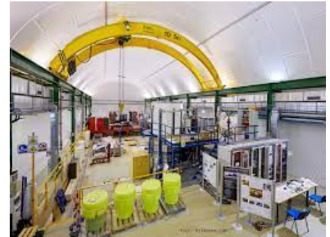
Figure 8.3: LSC Facilities at Canfranc (Spain). This underground laboratory is located below Tobazo peak, and was built expanding an old train tunnel between Spain and France. Currently it hosts several experiments for neutrino and dark matter search, among others.
